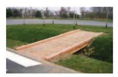
Made of treated Douglas fir or heart of Douglas fir, grooved planks 36 mm thick, fixed using stainless steel screws to a wooden backing strip.
