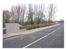
The wood & steel guardrail is bolted to the wall or the concrete barrier
