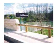
A steel device designed to connect our wood & steel guardrails TM18, T 18 & T 22 to all concrete walls. Pre-assembled component including 1 m long guardrail, powder coated end piece bolted to the wall, wooden spacer and standard fishplate TL 62
