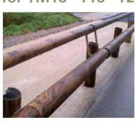
Powder coated steel device adaptable to all our wood & steel guardrails; with two off-set arms placed on fishplates hardware and a steel hoop to accommodate the 12 cm diameter half round wooden handrail.
