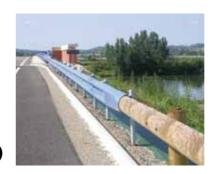
T.A.T. transition for TM18 - T18 - T22 to W beams and Euro ET end terminals.
