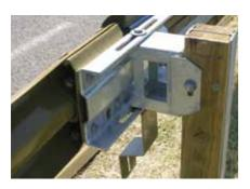
Steel device connecting the wood & steel T40 barrier with a standard W beam
