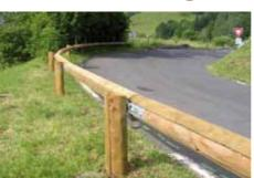
The C post planed wooden cover does slide inside post wings, giving to the spacer + post unit the appearance of a complete diameter 18 cm round log.
