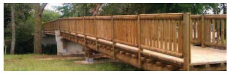
Solid Wood gangway. Structure made of logs of 10 - 12 and 28 cm  $\emptyset$ , dimensions according to Eurocode 5. Grooved wooden decking, 36 mm thick. Mixed Wood & Steel
