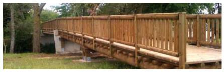
Solid Wood gangway. Structure made of logs of 10 – 12 and 28 cm Ø, dimensions according to Eurocode 5. Grooved wooden decking, 36 mm thick. Mixed Wood & Steel
