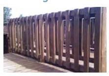
Planed posts 120 mm x 120 mm in 1.60m - Barrel panel: length 2.00 m, height 0.93 m, 10 planed barrels 80 mm x 30 mm, to be screwed on the posts. 2.00 m post spacing, height above ground of the barrels: 1.03 m, height above ground of the post: 1.03 m, ground clearance 0.10 m
