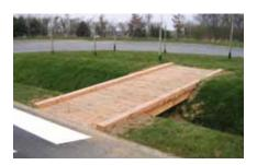
Made of treated Douglas fir or heart of Douglas fir, grooved planks 36 mm thick, fixed using stainless steel screws to a wooden backing strip.
