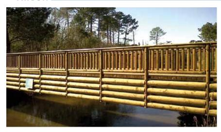
Straight mixed wood & steel gangway. Galvanized steel structure, dimensions according to Eurocode 3, wooden cladding. Grooved wooden decking, 50 or 80 mm thick. Mixed Wood & Steel Parapets
